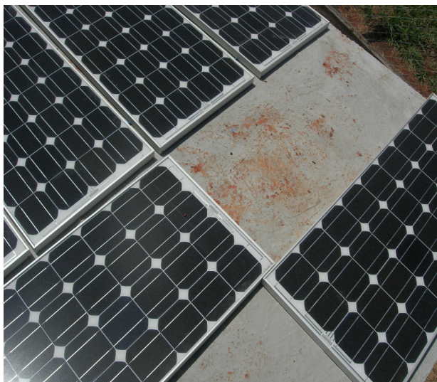
FIGURE 7: Position of the solar panels over the roof of the accommodation.
