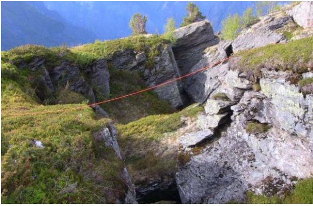
Fig. 6 - ERT cable crossing a large tension crack in the Joasete area
