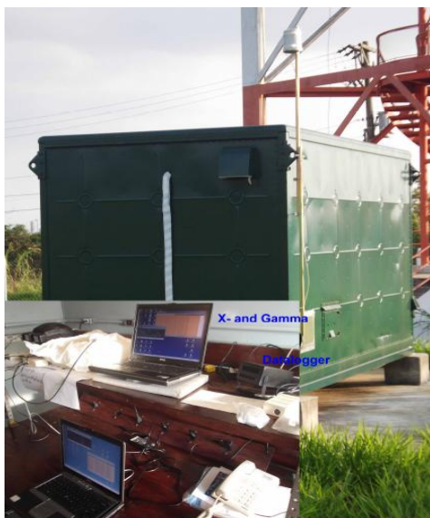
Figure 2: Trailer and instruments inside the trailer at the ACA Tower. Note the pluviometer at the top of the pole attached to the side of the container.
