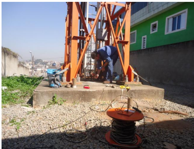
Photo 3 - PS test being performed in the telephone tower foundation.
