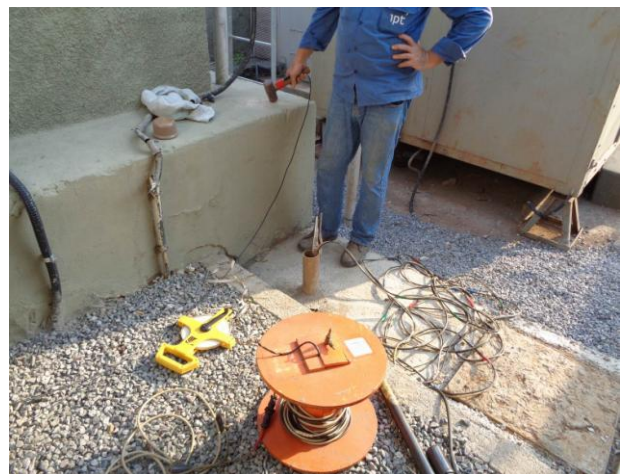
Figure 7 - PS test being performed in the telephone tower foundation.
