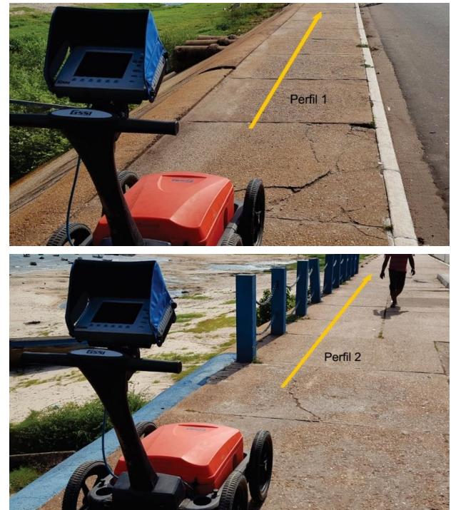
Figure 2 - Profiles 1 and 2, respectively, on concrete pipes and metal pipes
