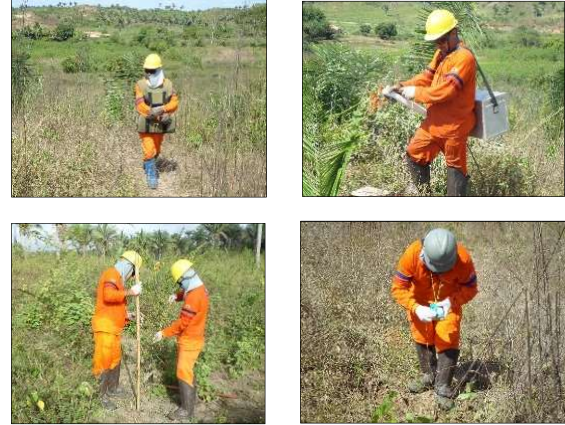
Figure 5: Loading - explosives transport, fuze transport and priming, tamping and galvanometer testing.
