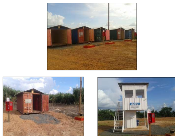
Figure 1. Mobile temporary storage with container - security box and separate storage locations for explosives and accessories.
