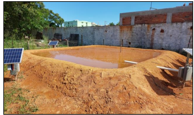
Figure 4 – The reduced-scale reservoir after the water filling-infiltration experiment
