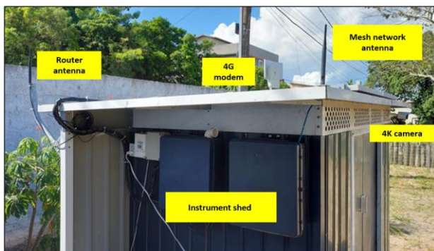
Figure 3 – Field instrument shed responsible for controlling the mesh network, storage and telemetry of microseismic data and filming of experiments
