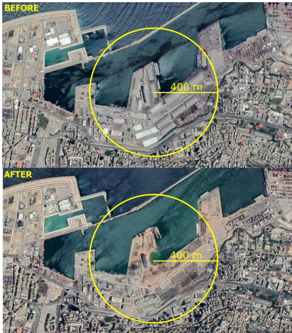
Figure 1 - Images before and after the explosion at the Beirut port. The destruction reached a radius of 400 meters from the explosion location.
