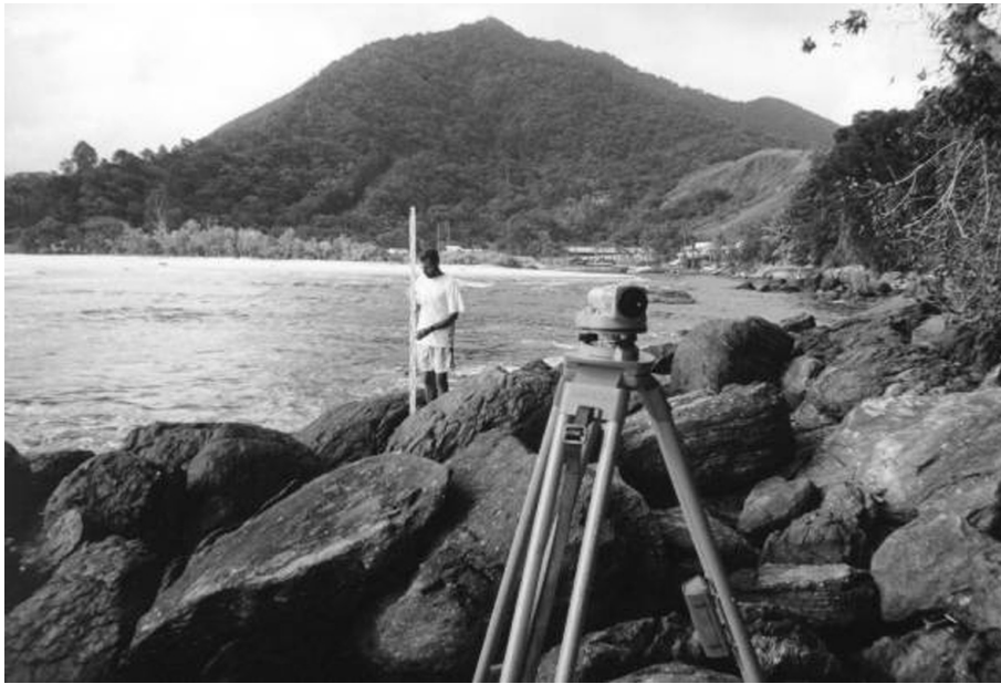
Figure 2 – Equipment N3 Wild with Mira Invar used to level Barra do Una. The survey was done with UNA1 and UNA2 stations georeferenced as base for measurement departure and arrival. The equipment used is a ZEIS Elta R50, precision 5" for angular and 5 \text{ mm} \pm 3 \text{ ppm} distance measurements. Linear precision reached was 1:18000.
