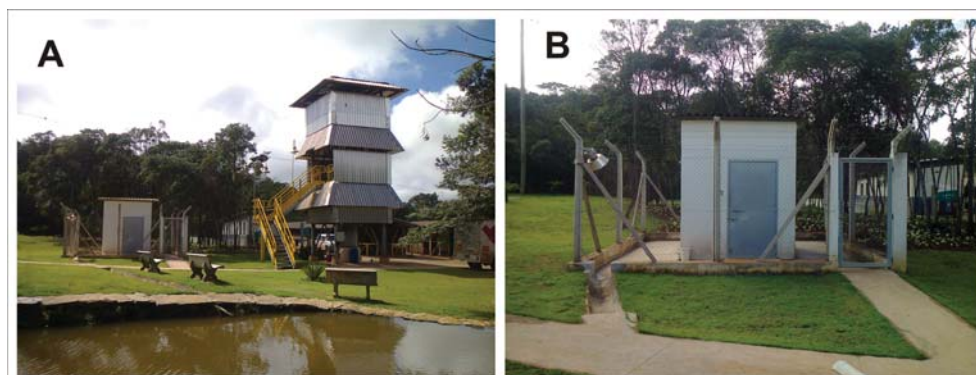
Figure 9 – Bunker for containment of radioactive source. (A) Localization of bunker in context of the Geophysical Well Logging Test Site; (B) Detail of bunker access.
