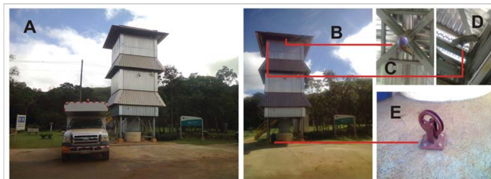
Figure 10 – Access and coupling system for vehicles and moving equipment. (A) Access to GWTF; (B) Positioning of cable pulley system; (C) Upper central pulley; (D) Upper support pulley; (E) Lower pulley.
